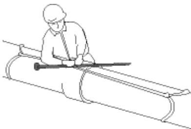
The spigot must be fully inserted to the full depth of the socket. The final 10% of spigot penetration is vital to the interference fit.
