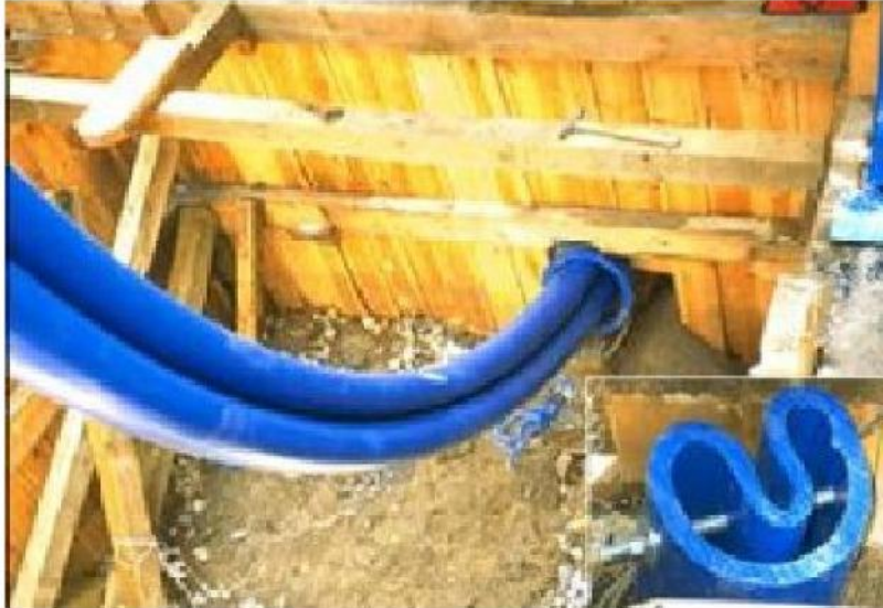
"Compact Pipe", insert showing cross-sectional shape - available from Iplex Pipelines
