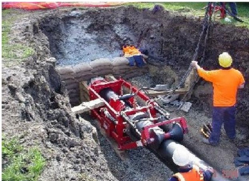
Swage lining DN500 showing reducing die and rollers, Hobart Tasmania (photo courtesy CLM Trenchless)
