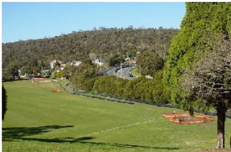
Butt welded PE pipes ready to be used – photo courtesy of CLM Trenchless
